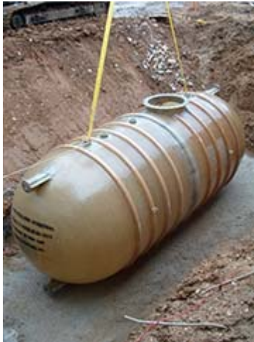
Rainwater collection system
